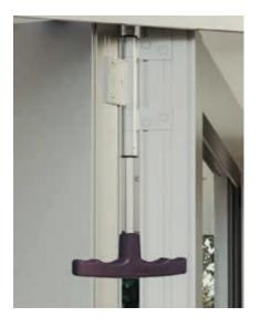
STEP 2 From the outside use the included Tomma T Bar to rotate the adjusting screw either clockwise for up or anticlockwise for down. One turn = 1.0mm
