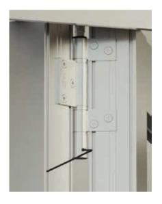
STEP 1 Loosen the locking screw by rotating anticlockwise for 2 turns (720deg)
